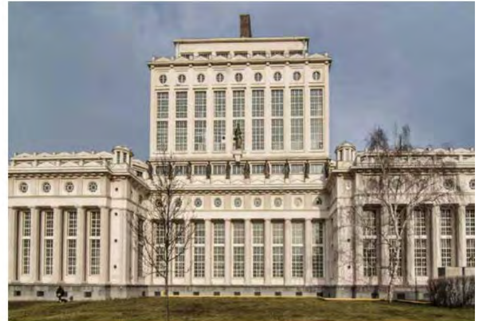
The magnificent neoclassical design of the Prague-Podolí treatment plant emphasizes the importance to the city of its water-supply system. (Wikipedia Commons)
